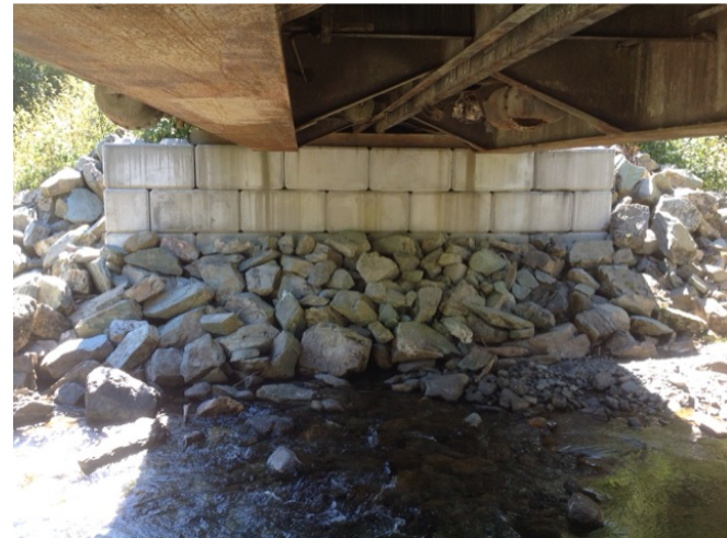
Right Bank Abutment when facing downstream
