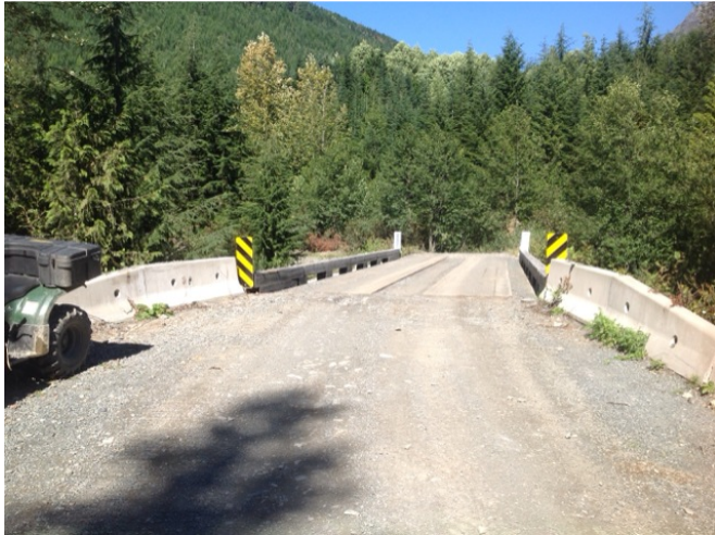
Approach from Right Bank when facing downstream
