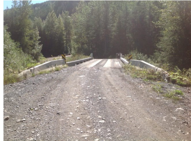
Approach from Left Bank when facing downstream
