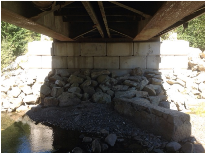
Left Bank Abutment when facing downstream
